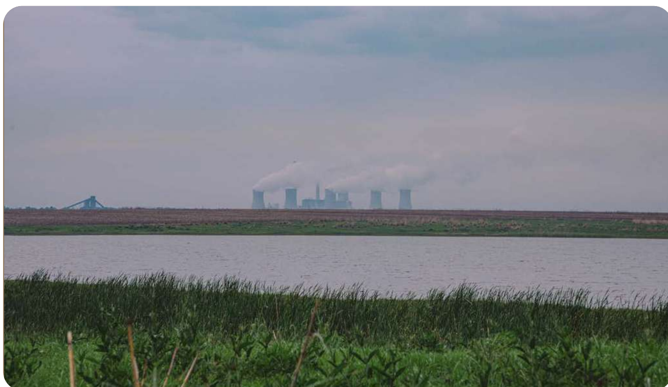
Matla pollution control dam
